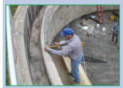
The outdoor waste water tanks were originally constructed in 1939, and no repairs had been made in almost 20 years. Corroding and spalled areas, as well as exposed rebar had to be repaired.
